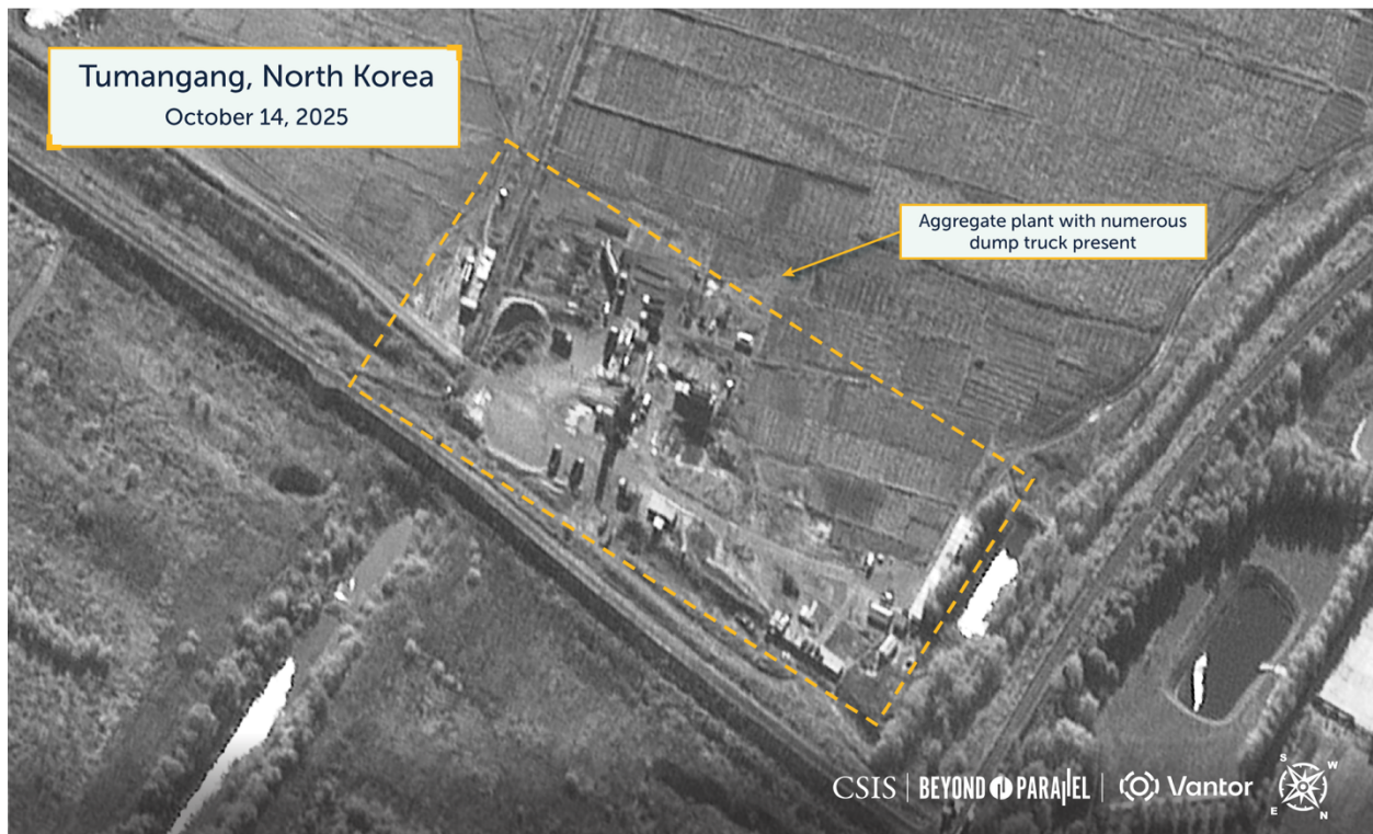
The temporary aggregate plant supporting North Korea's bridge construction effort, October 14, 2025. Copyright © 2025 by Vantor. Image may not be republished without permission. Please contact imagery@csis.org .
