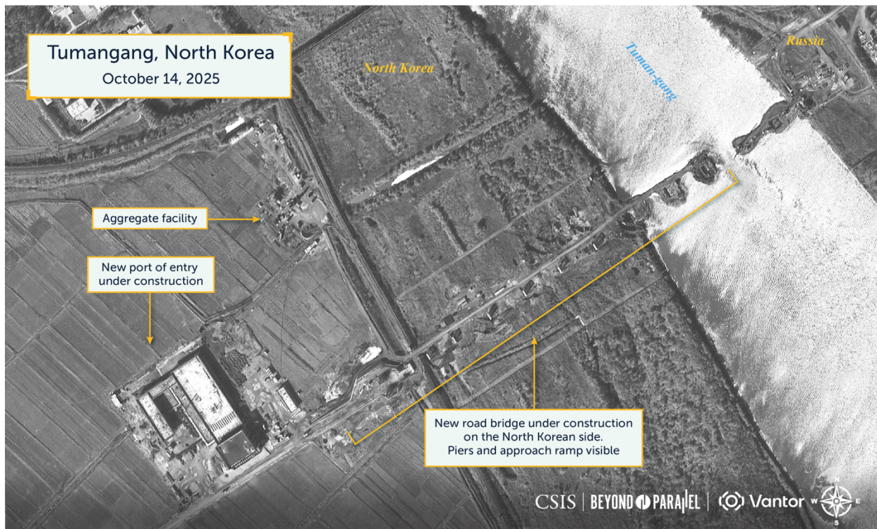
Construction activity on the North Korean side of the Tumangang to Khasan road bridge construction site, October 14, 2025. Copyright © 2025 by Vantor. Image may not be republished without permission. Please contact imagery@csis.org .
