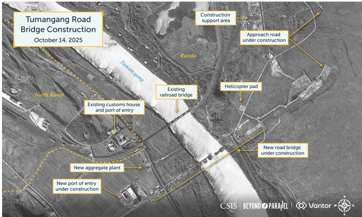
An overview of the Tumangang to Khasan road bridge construction sites, October 14, 2025. Copyright © 2025 by Vantor. Image may not be republished without permission. Please contact imagery@csis.org .
