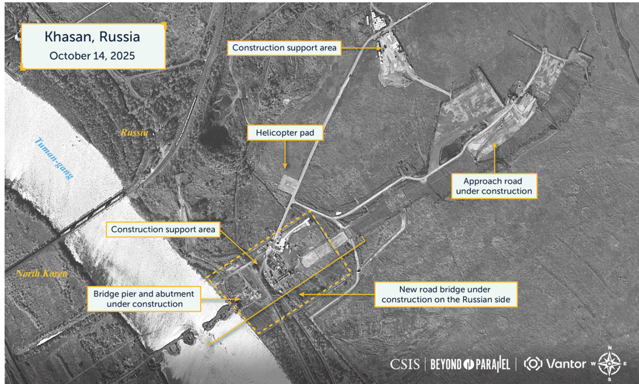
Construction activity on the Russian side of the Tumangang to Khasan road bridge construction site, October 14, 2025. Copyright © 2025 by Vantor. Image may not be republished without permission. Please contact imagery@csis.org .
